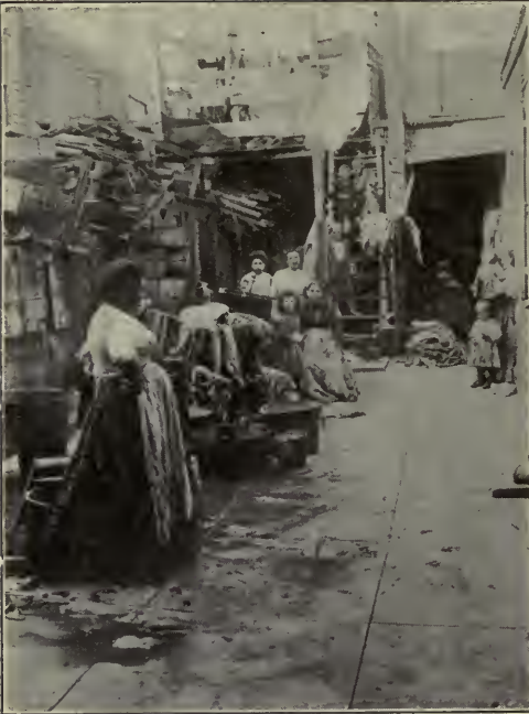
A COURT CONTAINING 3 WATER CLOSETS AND 2 HYDRANTS, USED BY 13 FAMILIES COMPRISING ABOUT 60 PERSONS
